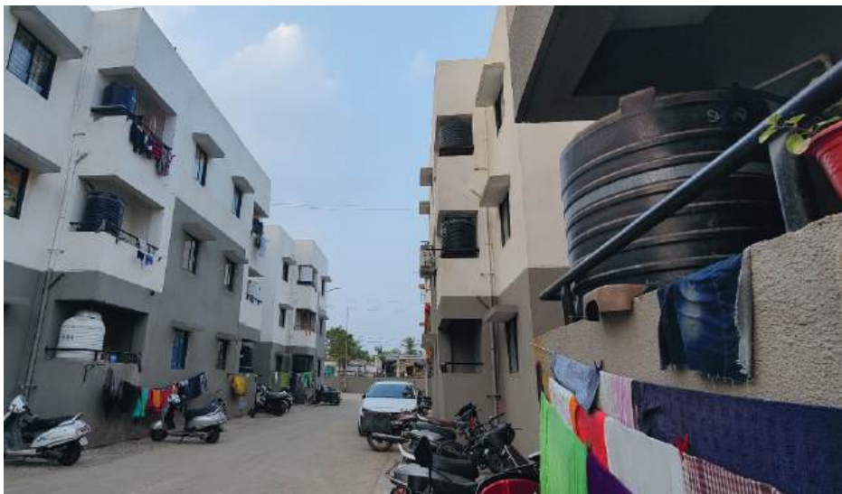
Photograph 11: The residents of Bhuj have installed water tanks at every household due to an intermittent water supply. Installing such water tanks causes uneven water consumption, impacting distribution networks and hence is not advisable, this issue is not unknown to government authorities. The municipalities in both cities are aware of such techniques employed by citizens to bridge the system inadequacies.
