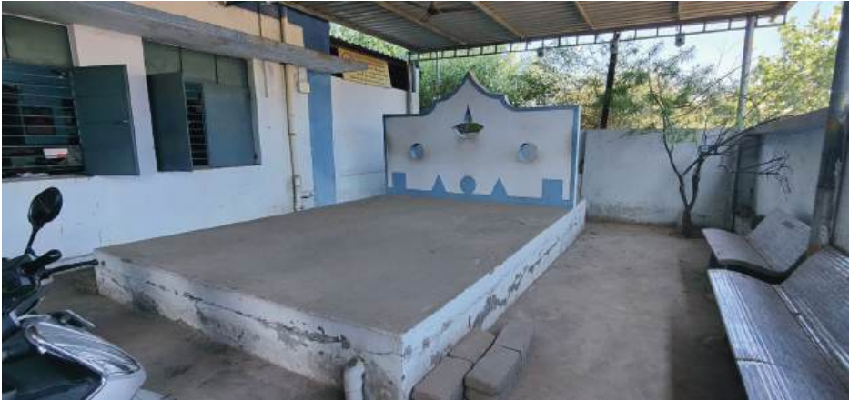
Photograph 12: Rainwater harvesting tank doubling up as a performance stage in a school
